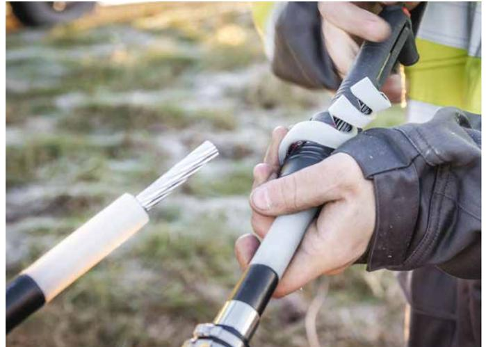
Ensto ST280 is designed to chamfer the primary insulation near the connector or lug in MV cables. This provides a smooth transition from insulation to connector or lug for the accessories installed. The application range  $\varnothing$  is 15-60 mm and the chamfer is 45°.
