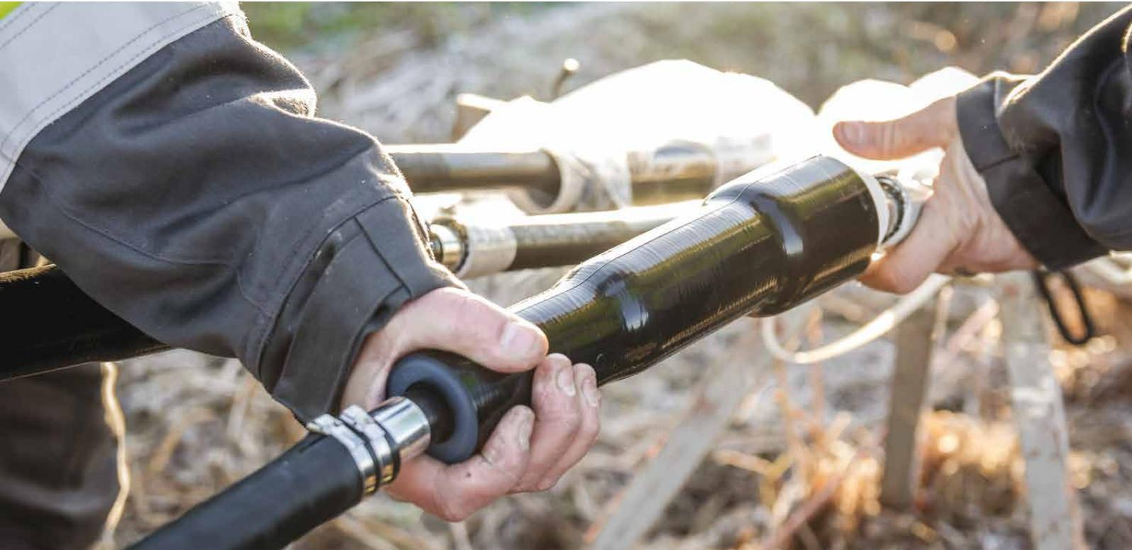
The reliability of several components integrated into one body and shorter installation times are the main advantages of cold-shrink and hybrid technologies.
