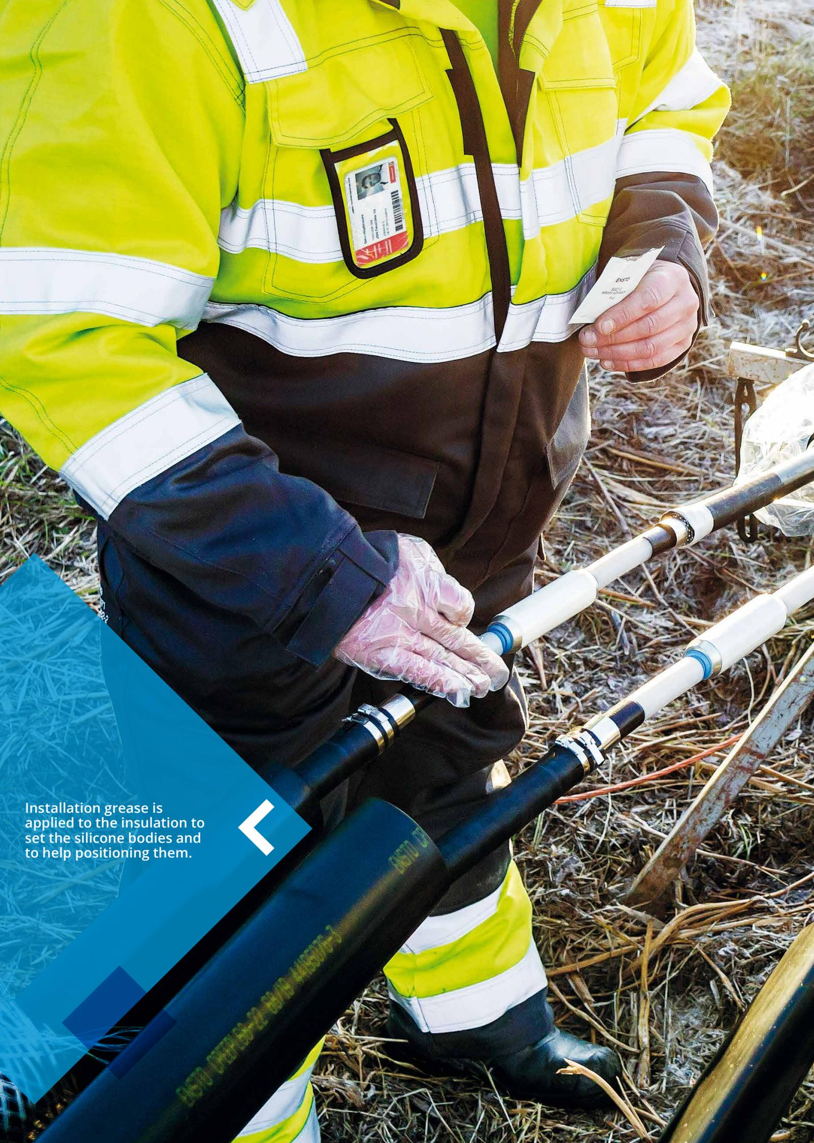
Installation grease is applied to the insulation to set the silicone bodies and to help positioning them.
