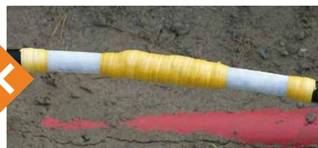
Stress control and sealing mastics are sensitive to heat and melt when the tubes are heated.
