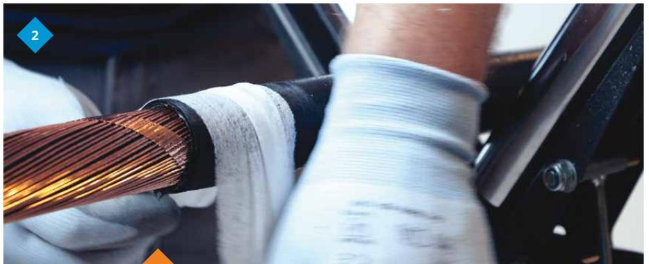
Always clean the outer sheath before removal and after grinding it.
