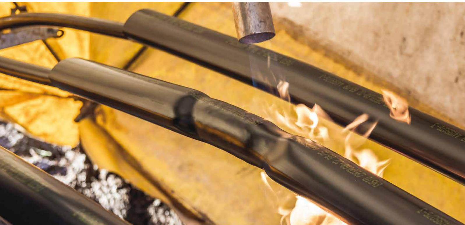
The mechanical robustness of heat-shrink accessories is the main advantage of the technology.
